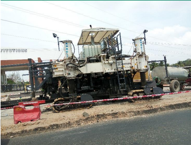
Exhibit 6: Site progress – Cement paver
