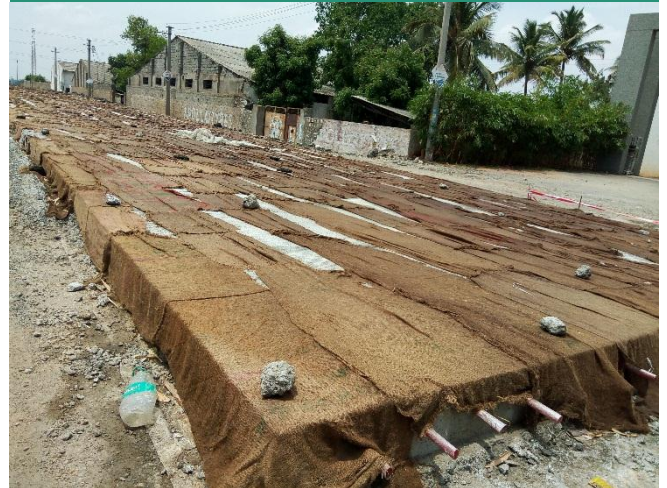
Exhibit 7: Site progress – Curing
