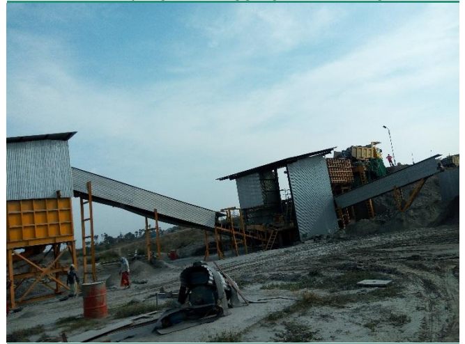
Exhibit 5: Site progress - Aggregate Crushing
