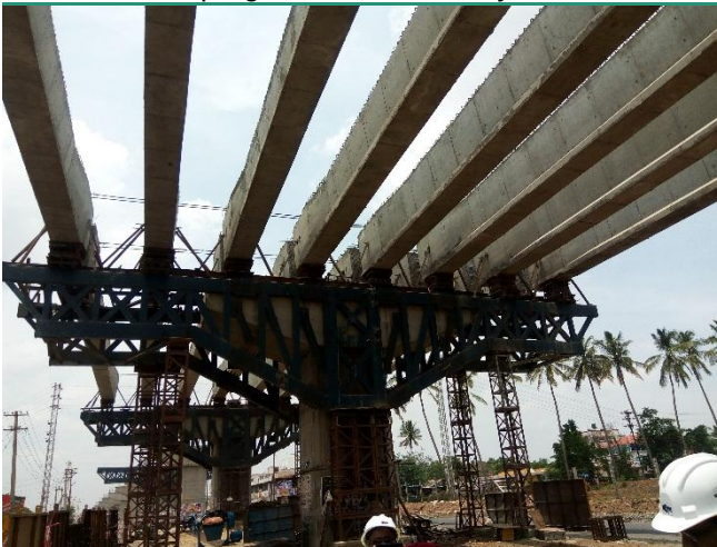
Exhibit 8: Site progress – Elevated Flyover
