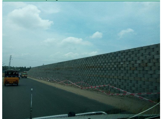
Exhibit 9: Site progress – RE Wall
