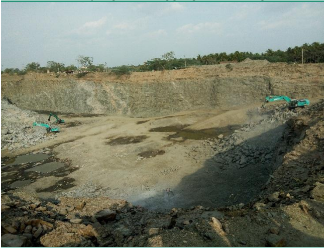
Exhibit 4: Site progress - Aggregates Mining
