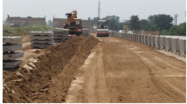
Fig 26 – A flyover in the making
