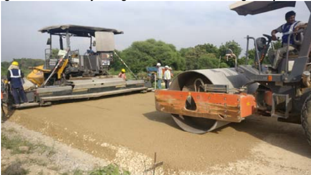
Fig 27 – The freshly laid granular sub-base being compacted
