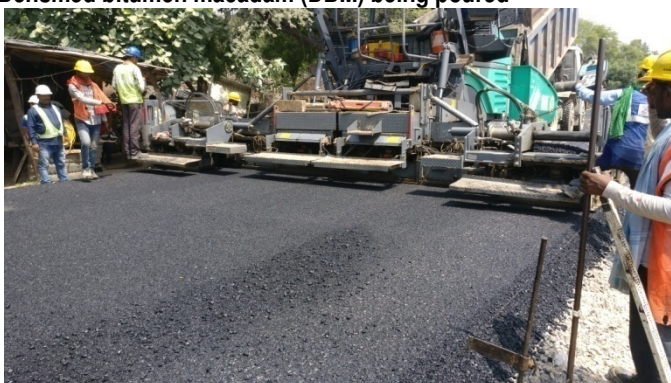
Fig 24 – Densified bitumen macadam (DBM) being poured
