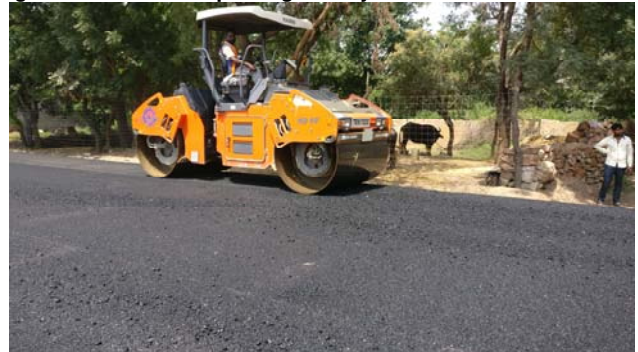
Fig 28 – A roller compacting freshly-laid DBM
