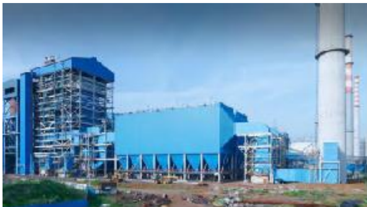
Chart 9: ESP, 180MW coal-based power plant for OPG Power, India
