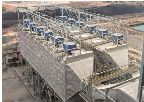
Chart 10: ESP, power plant for Bhubaneswar Power, India
