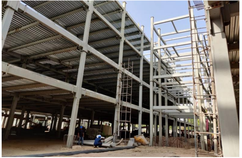
Exhibit 2: Construction work at GTB Hospital in full-swing
