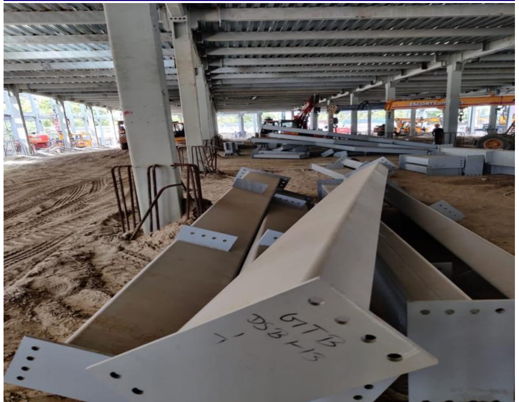
Exhibit 3: Construction work at GTB Hospital in full-swing
