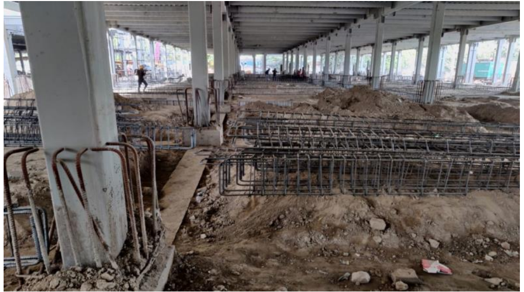
Exhibit 4: Construction work at GTB Hospital in full-swing
