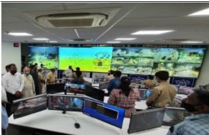
Exhibit 15: Command & control center at Aurangabad
