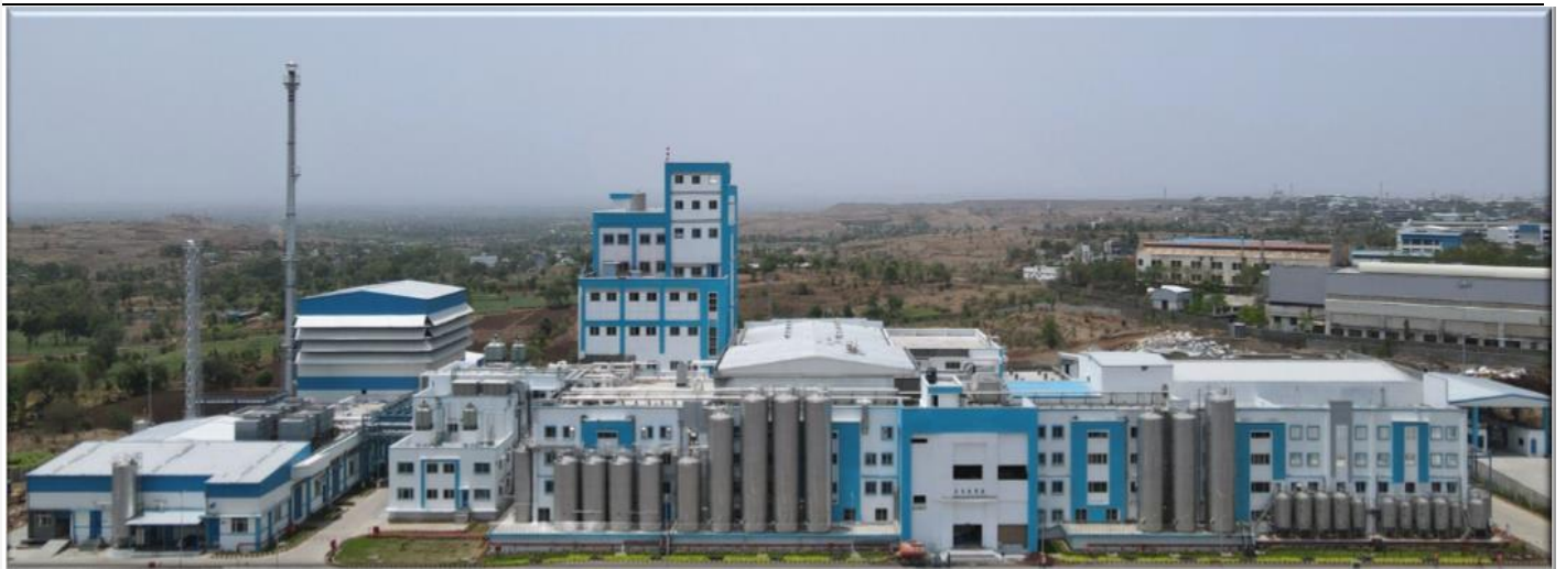
Exhibit 8: Ranjangoan Dairy factory commercialized; Cheese line to be commissioned in FY24
