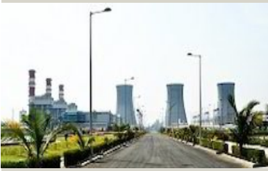
DGEN Gas Plant (1200MW) Dahej, Gujarat
