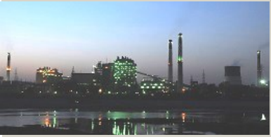
AMGEN Coal Plant (362MW), Ahmedabad, Gujarat
