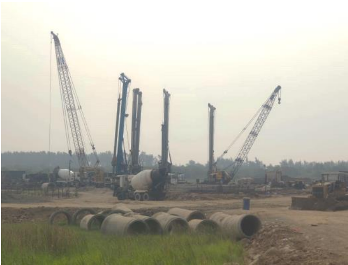
Exhibit 11: Excavation in progress at SBR Vasai
