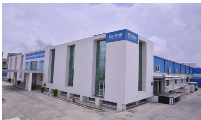
Exhibit 37: GPIL's Jaipur smart metering facility
