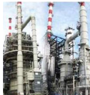
Re-boilers / Hot Oil Heaters
