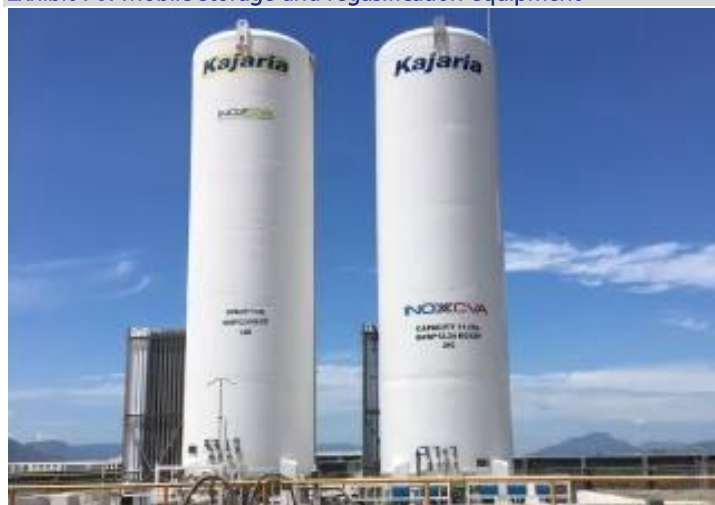
Exhibit 76. Mobile storage and regasification equipment
